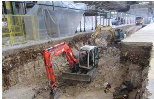
Fig.1: Santier in lucru
